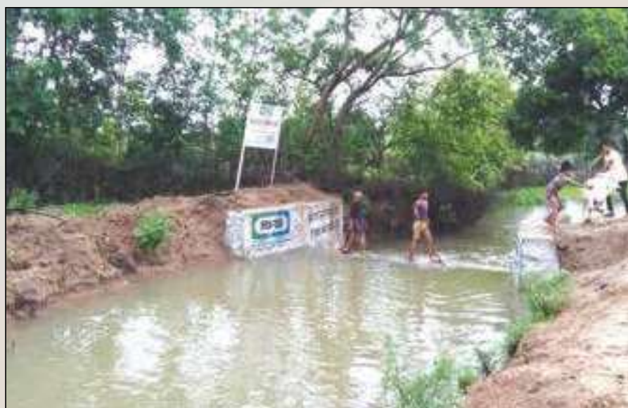
Check dam constructed in village Bilhani, District Sagar (Madhya Pradesh) under IFFCO-Tokio Integrated Rural Development Project- Bundelkhand
